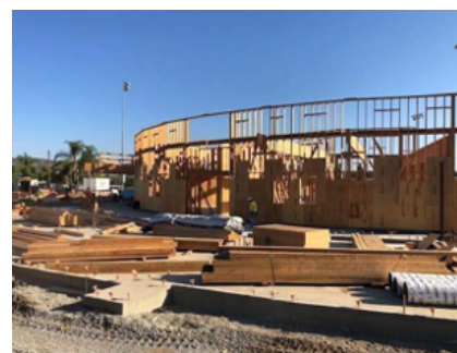
CONSTRUCTION OF CHET F. HARRITT CLASSROOM ADDITION
